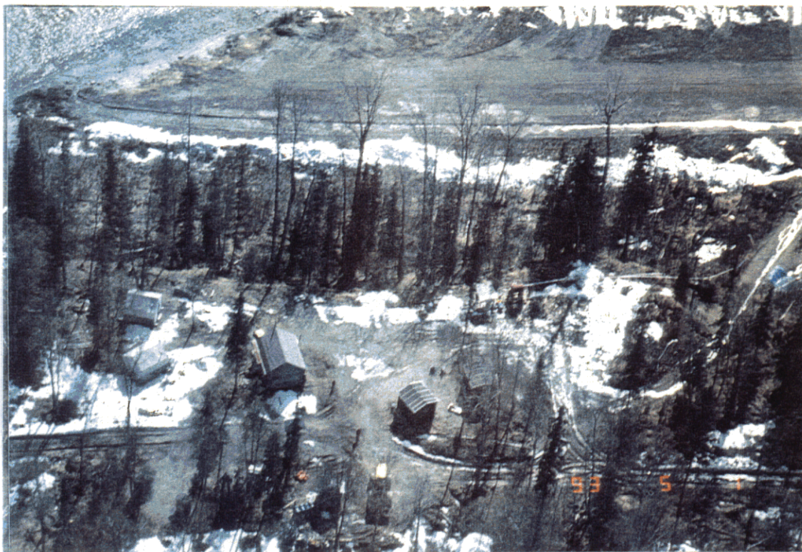
Camp - large cookhouse is in good condition.
