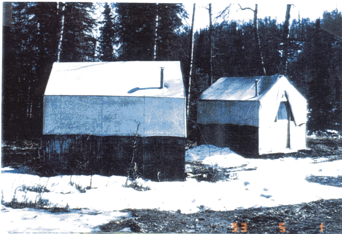
Four bunkhouses are good inside but need new paper outside.
