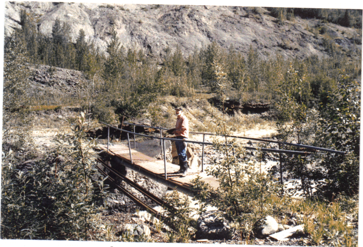
One of two foot bridges over Dan Creek
